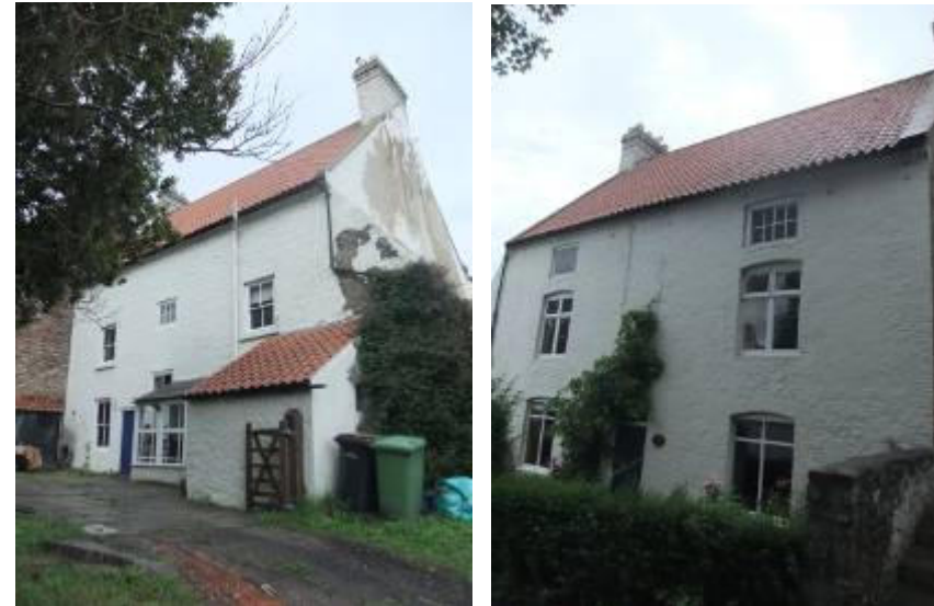
No. 1 Front Street has suffered from a considerable loss of historic character but the distinctive signs of a bread oven in the west facing gable end is a reminder of an older building
