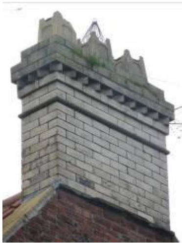
19th century chimney pot with brick detailing
