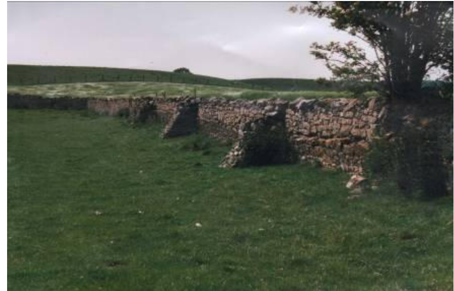
Remains of the deer park wall. This stretch is clearly in two phases, presumably the deer park wall has been lowered and rebuilt over the centuries (photo: John Smith, Bishop Middleham)
