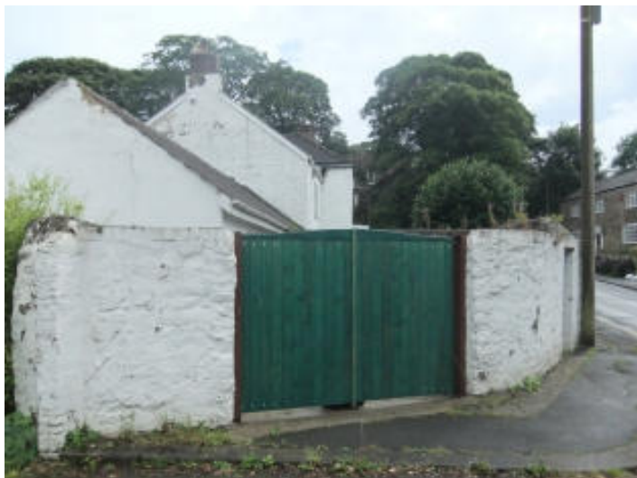
Example of limestone walling
